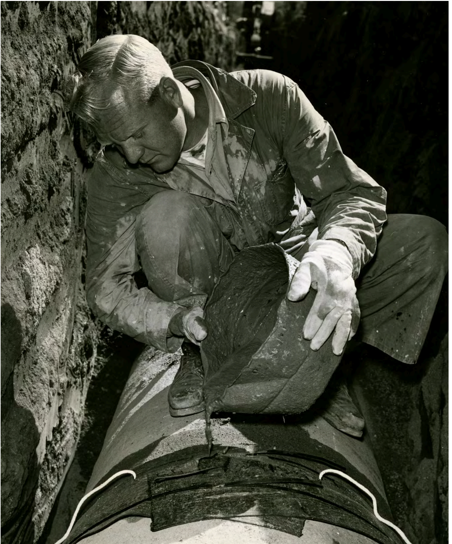
▲ The District's Coast Supply Line is a 27-inch pipeline that transports water from the Metropolitan Water District of Southern California's Diemer Filtration Plant to the District and to South Coast Water District. In this undated historical photo, a District employee repairs the exterior concrete coating of a section of the welded steel pipe.
