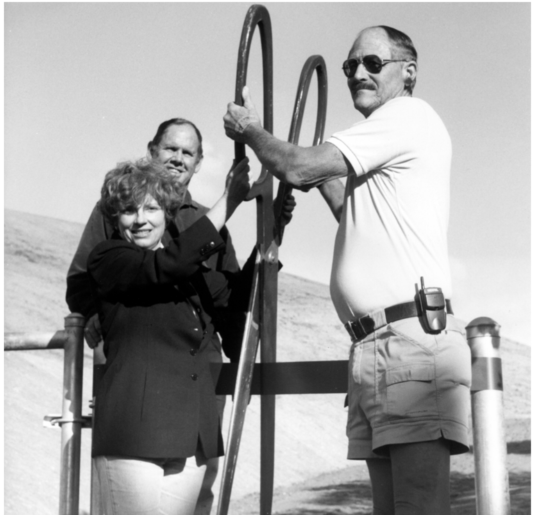
▲ In 2000, the District finished the construction and filling of our Zitnik Reservoir, which provides five million gallons of emergency storage for fire protection in North Laguna. In addition to completing this integral part of our water storage system, the District dedicated the Thomas Cummings Coastal Wilderness Park Access Point to Laguna Coast Wilderness Park. Pictured from left to right is Board member Toni Iseman, Commissioner J.J. Gasparotti and Commission Chairman Bruce Scherer.
